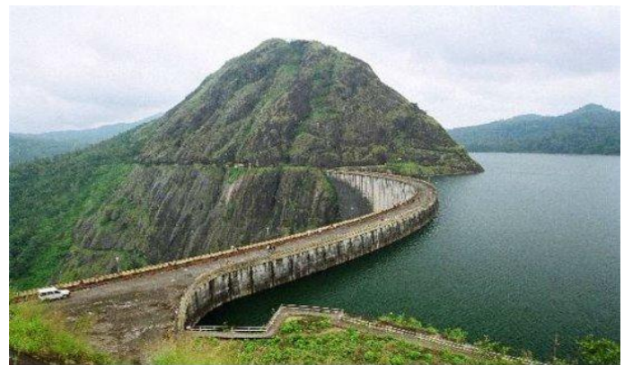
Fig -3: Upstream view of Idukki dam
