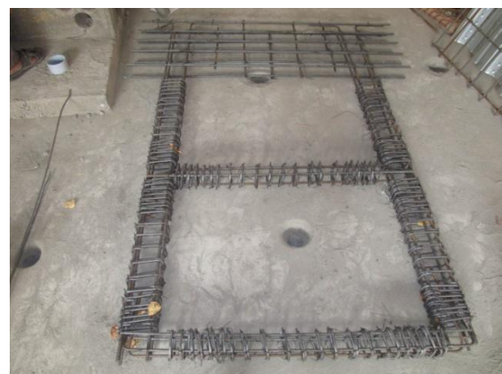
Fig-2: Reinforcement Grill for the RC Frame
