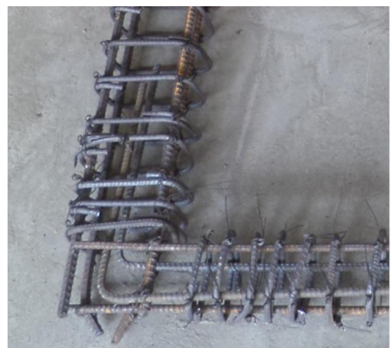
Fig-3: Closer View of Beam-Column
