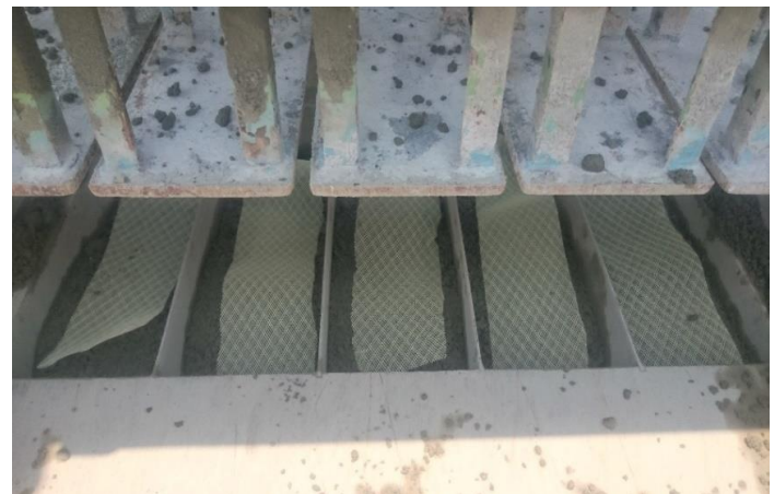
Fig -1: Placing of Geo Grid Mesh in between the Concrete Blocks
