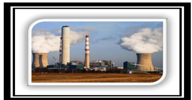
Figure: Self-Supporting Steel Chimney
