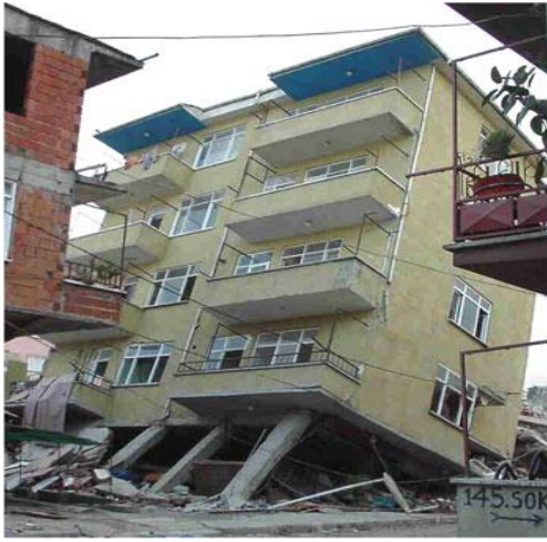
fig 3(c)Ground soft storeyfailure fig 3(d) soft storey failure pattern
