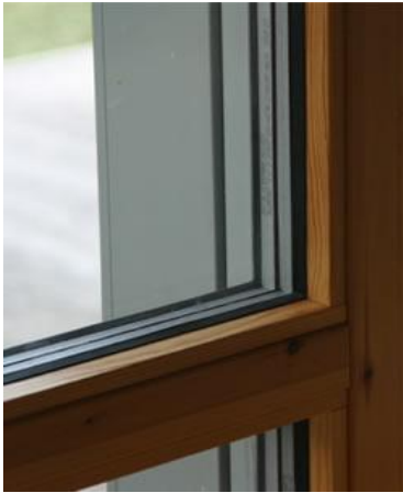
Fig: 9 Triple Glazed Window
