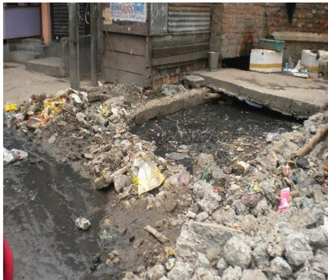
**Figure-11:** Open and clogged drain
