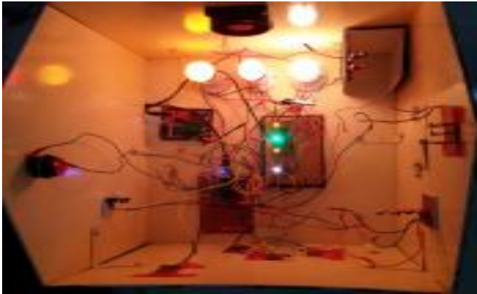
Fig-4: Controlling of appliances
