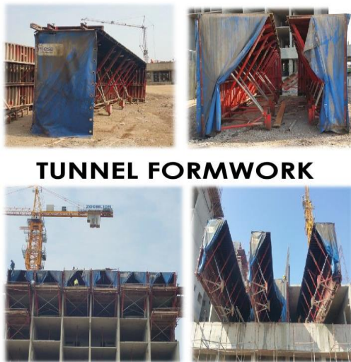
Fig - 1: TUNNEL FORMWORK
