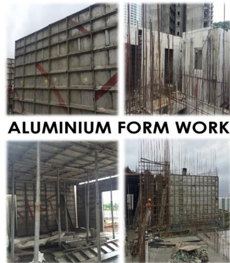
Fig - 2: ALUMINIUM FORMWORK
