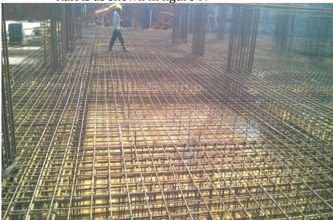
Fig-9: Raft Foundation
