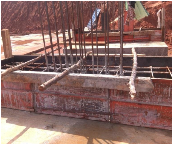
Fig-8: Combined Footing
