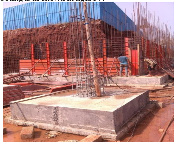
Fig-7: Isolated Footing
