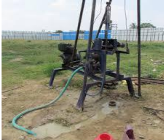
Fig-3: Plate Load Test
