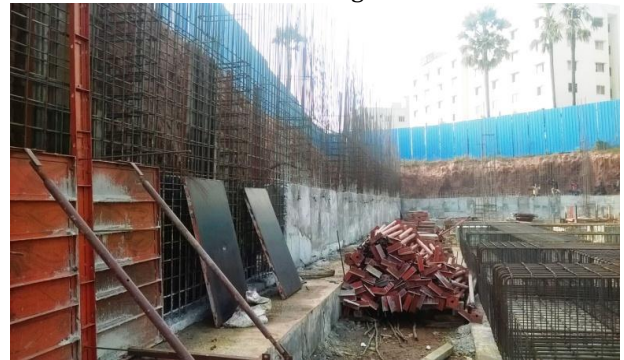
Fig-6: Retaining Wall
