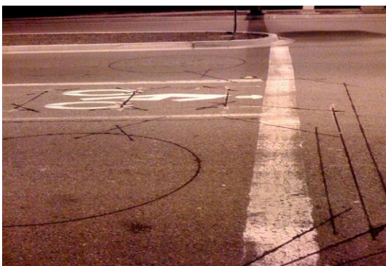
Fig -1: Inductance loop installed in the road for Cars and bikes.
