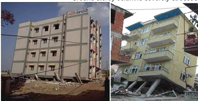
Fig -3: failure due to large lateral displacement in soft storey
