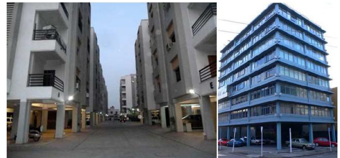
Fig -1: Soft storey in reinforced concrete buildings
