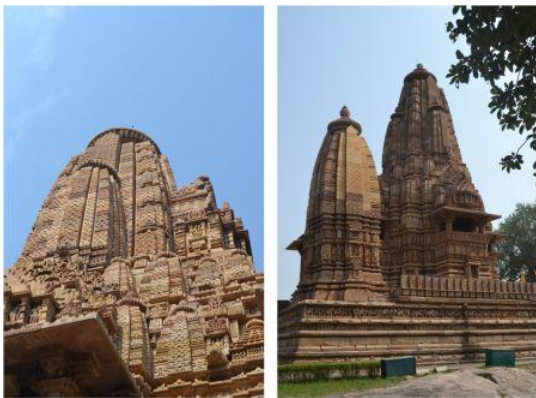
Picture 3: The whole structure seems to be integrated through the shikhara curve pointing towards the common axis
