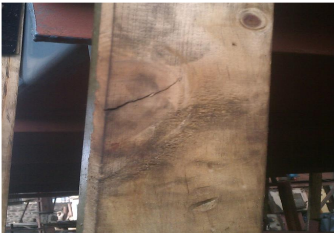
Fig-1.2: Failure Cause by Tension in Wooden Plank Assembly
