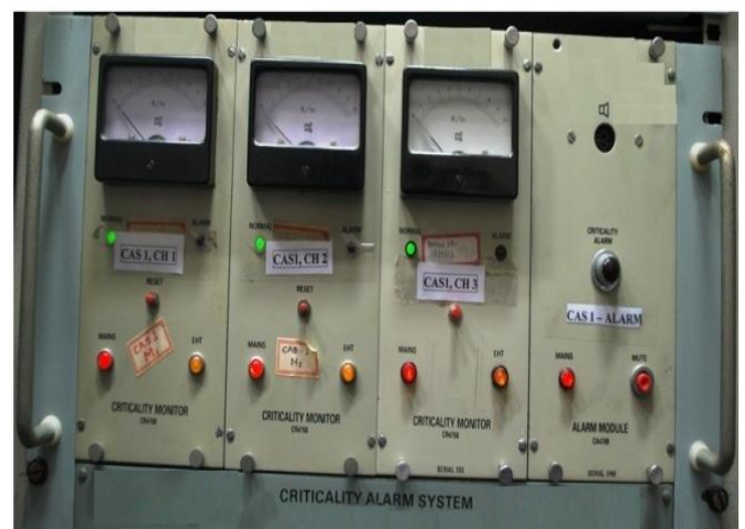
Fig 4: CAS unit consist of 3 Channels Alarm Module
