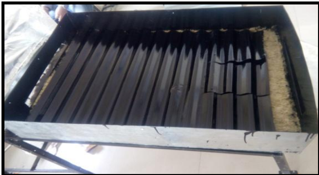
Fig - 6: Construction of flat plate collector
