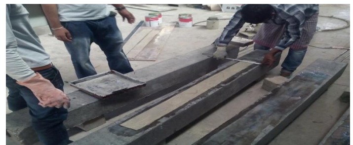
FIG 3: Strengthening of Beams by NSFRP Composites
