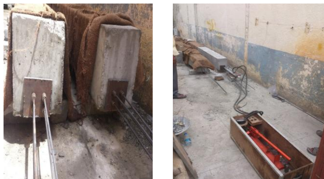
FIG 2: Post Tensioning of Beam
