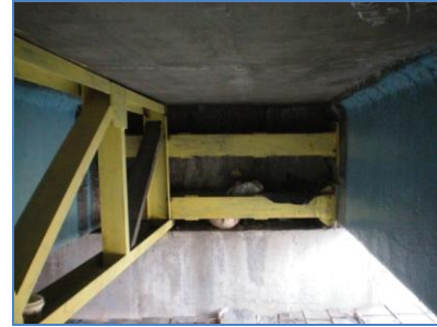
Connection of truss over main beam
