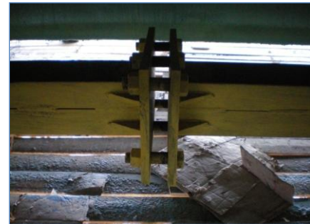
Pre-stressing Mechanism in Truss
