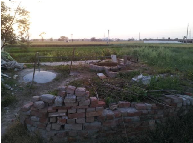
Fig -1: Septic tank investigated in the study
