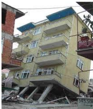
Fig -1.1: Collapsed Soft Storey Building from Earthquake
