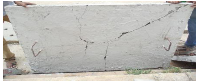
Fig-3.3: Typical crack pattern on compression side
