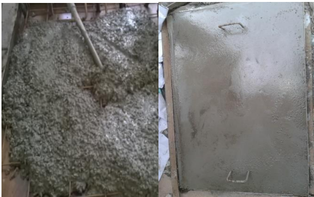
Fig -2.3: Casting, compaction and finishing of slab
