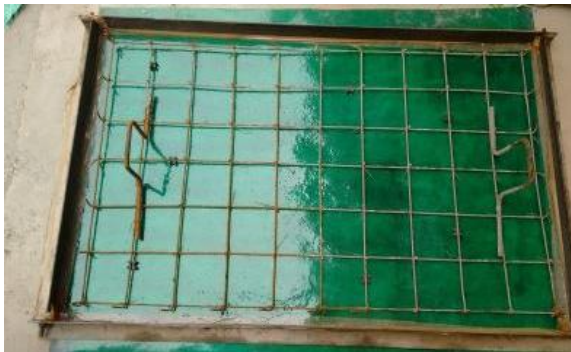
Fig-2.1: Typical reinforcement cages of a slab
