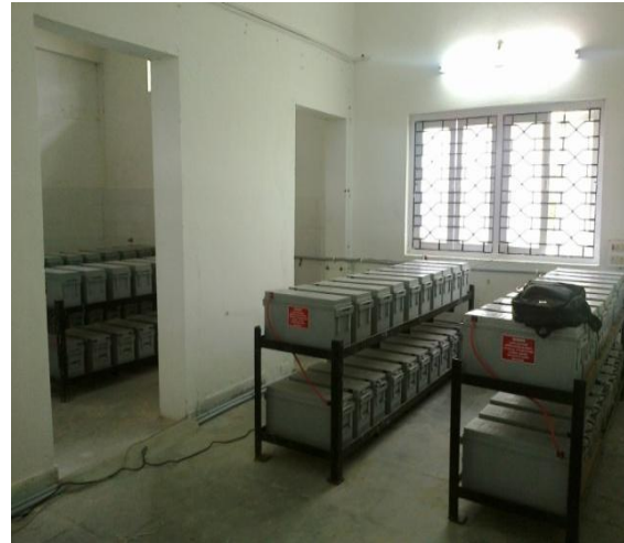
Fig.5: Solar Batteries
