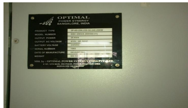
Fig: 4: Power controlling unit details
