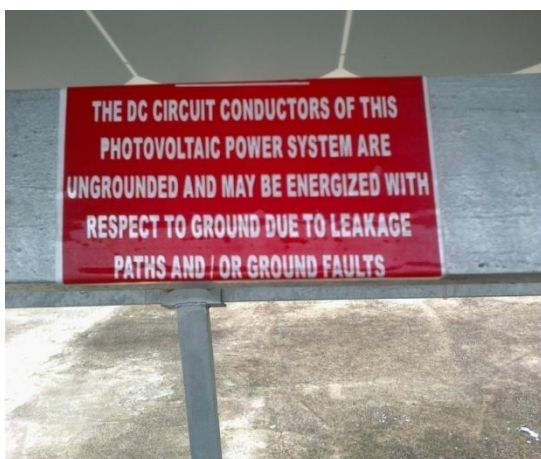
Fig.2.c: Details of Solar panels
