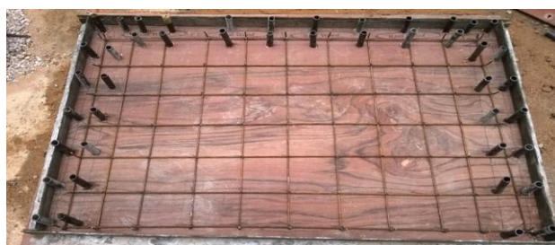
Fig -3: Mold for casting slabs.
