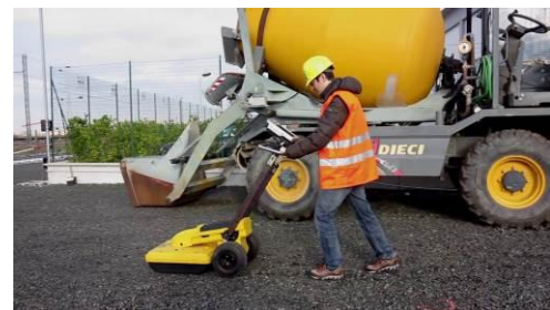
Fig.8: Ground Penetrating Radar System (GPRS)
