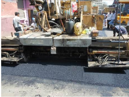
Fig.1: Unchecked Asphalt Paver Machine
