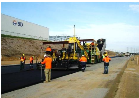
Fig.6: Laser based system used for road construction in Asphalt paver machine used in developed countries
