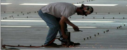
Fig 2: Installation of Shear Studs
