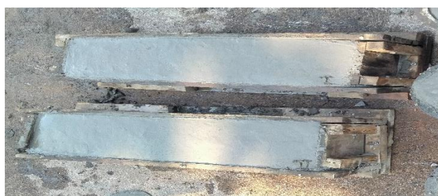
Fig-3: Casting of Cylinder, Cube & Beam.
