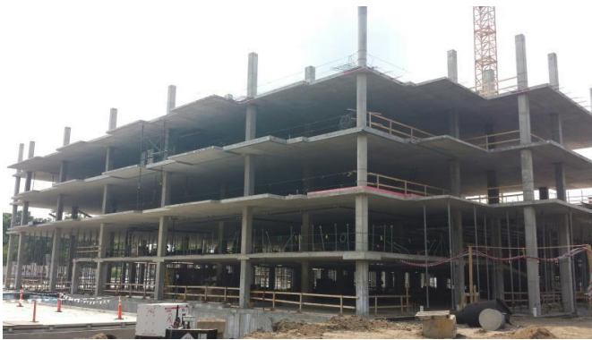
Figure-1: RC Frame Structure.
