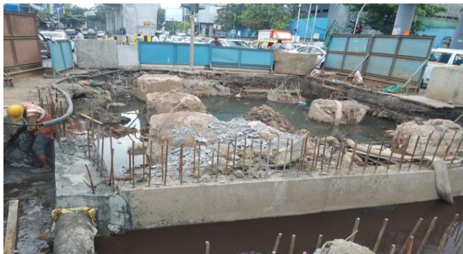
Fig -3: Utility drainage diversion slab at pile cap.
