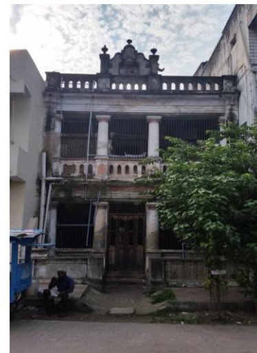
Fig -1: Karneeshwar kovil street house
