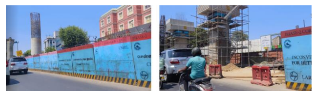
Figure 4 KV Metro Construction Site
