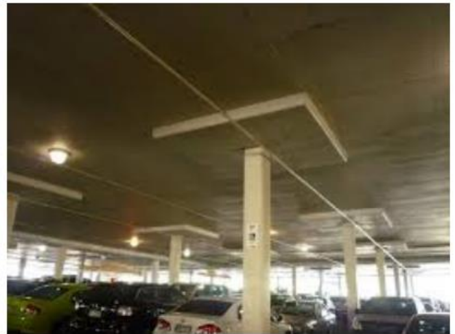
Figure 3: Aesthetic appearance of flat slab floor [4]
