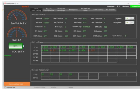
Fig – 4 : BMS data observation in PC master
