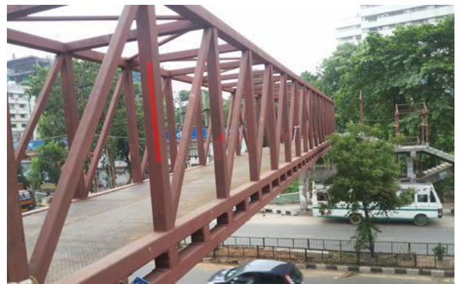
Fig. No. 1. Lattice Type Truss Pedestrian Bridge
