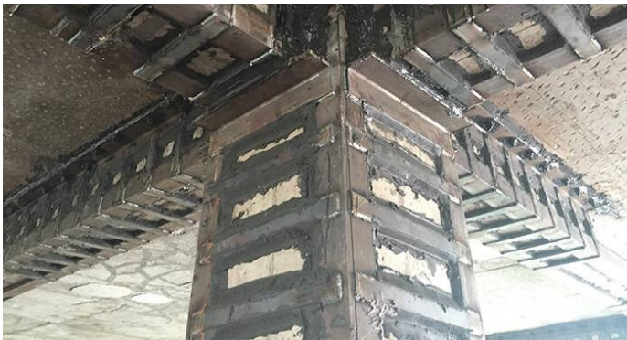
Figure-1: Concept of Jacketing
