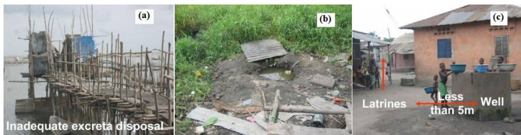
Figure 2. Water supply sources and their environmental implications in Cotonou: (a) Insufficient waste disposal on Lake Nokoue; (b) Water supply source pollution; and (c) Inadequate separation between pit latrine and well, as per the current WHO guidelines (15 m). Source: Totin et al.[17]
