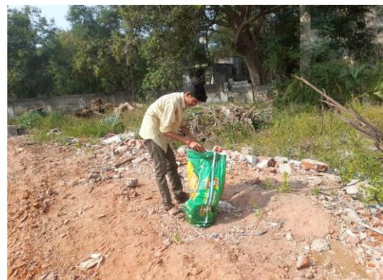
Fig3: Collection of RCA From Jntuk Dismantled Building
