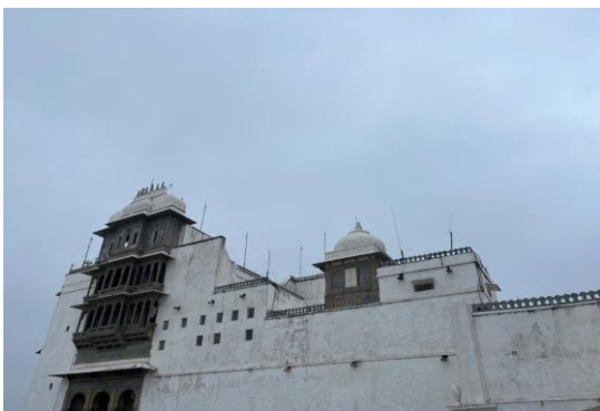
Fig.11 lime plaster on wall surface
