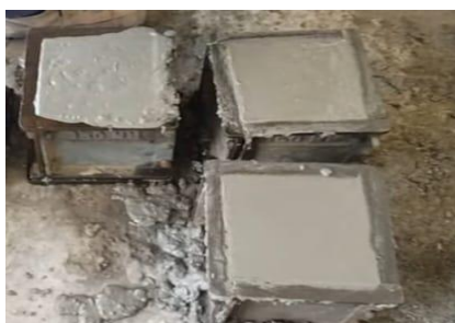
Fig. 13 Moulding of Concrete cube specimen
