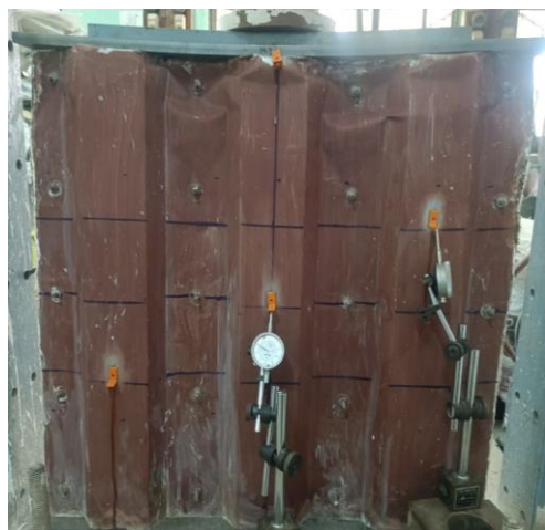
Fig. 5: Bulging of Sheet in between the Studs
