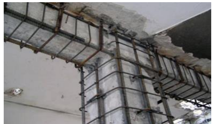
Figure 2: Reinforcing existing column
