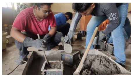
Fig.9 Placing and compacting the freshly concrete in moulds
