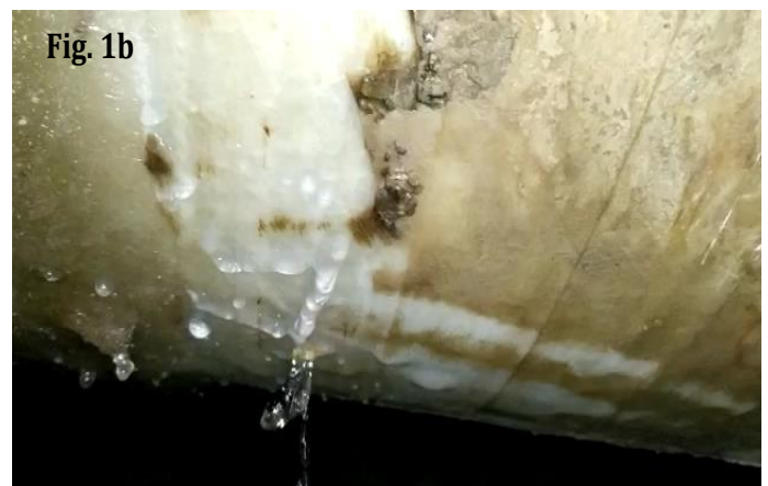
Fig.1a: Leakage through main pipe body; Fig.1b: Seepage through main pipe body
