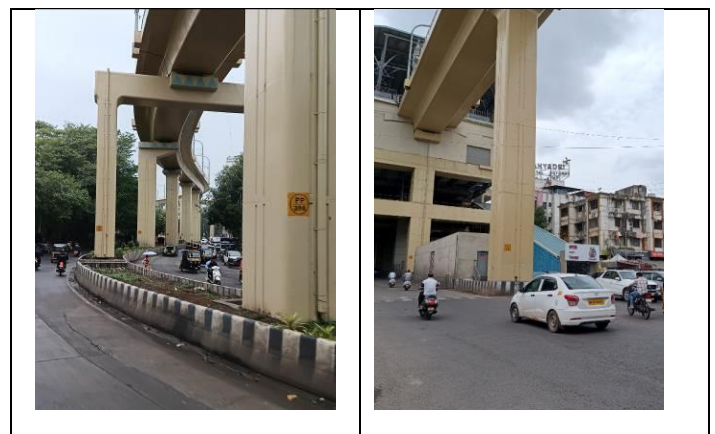
Fig 3: The continuous medians with relief breaks for crossovers for pedestrians to access residential areas on either side of the roads.
