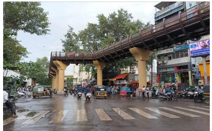
Fig 8: The skywalk for pedestrians to access the Metro station.
