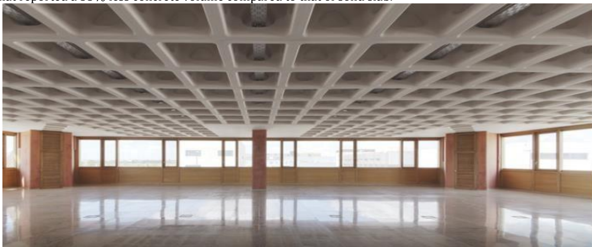
Figure 3 : Waffled floor slabs [3]
