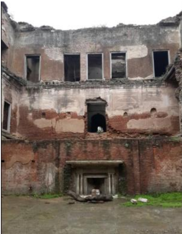
Figure 21 One of the broken sides of quila Androoni Quila, showing different materials of construction
