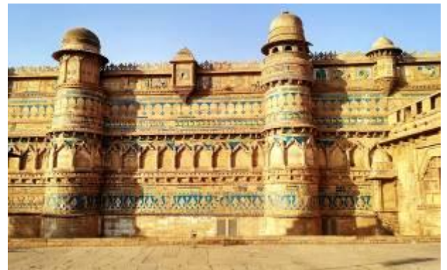
Figure 10 Exterior facade of Man Mandir Palace with coloured tiles used for decorations (Source- http://anarchytect.blogspot.in/2013/01/gwalior-man-mandir-palace.html , accessed on 4th April 2018)
