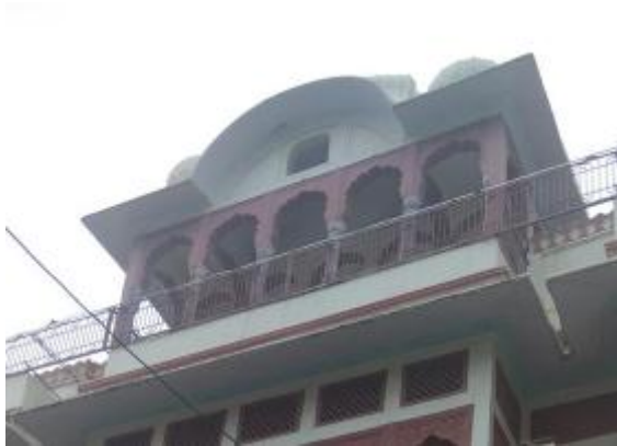
Figure 27 Bangladhar roof at entrance gateway of Bohra Kunj
