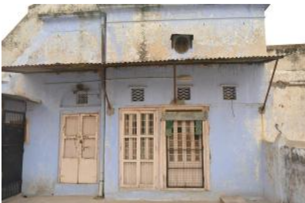
Figure 32 View of room added later on terrace with different architectural vocabulary
