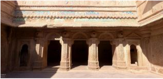
Figure 7 View of one of sides of courtyard in Man Mandir Palace showing the massive columns along with arches supported with beams, a combination of architectural construction systems (Source- Google Earth)
