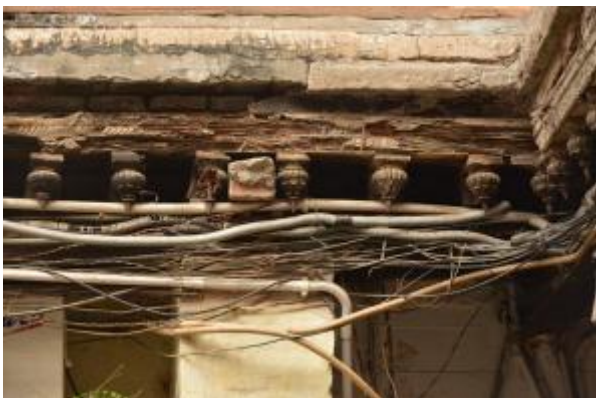
Figure 31 Timber beams used in Haveli
