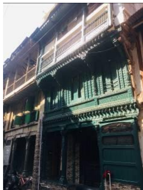
Figure 17 Front facade of one of the pol houses, Ahmedabad
