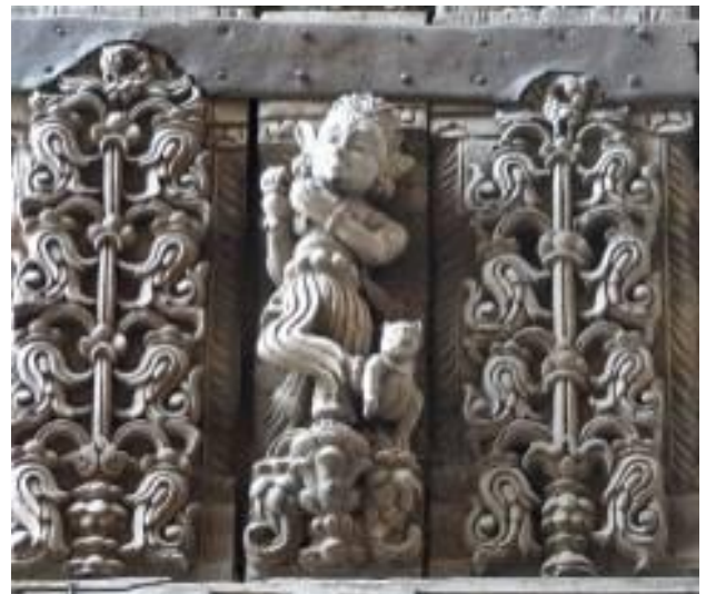
Figure 16 Carving in one of Pol house facades showing Lord Krishna —faith of locals (Source: Ahmedabad Municipal Corporation, World Heritage Nomination Dossier - Historic City of Ahmadabad, 2016, UNESCO)
