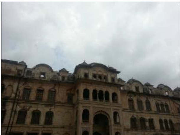
Figure 22 Gateway and front facade of Quila Androoni
