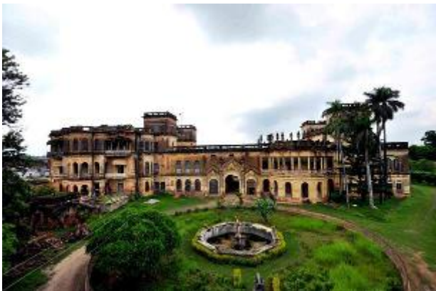
Figure 35 Side view of Kothi, from eastern side, showing the central passage for vehicles
