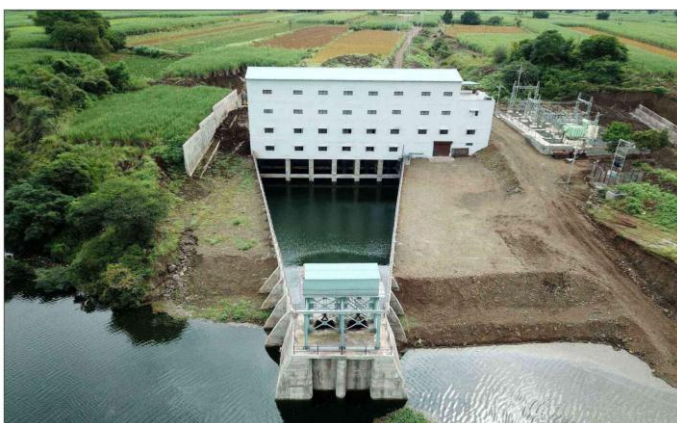
LIS Pump House Photo
