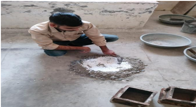
Fig -1 Mixing of EPS BEADS in concrete
