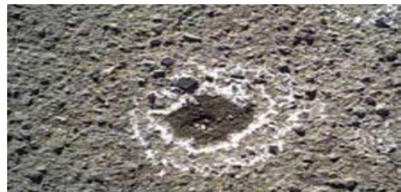
Fig-1: A burst salt blisters
