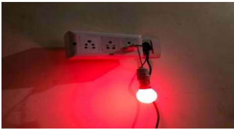
Fig -3: smart switch on condition
