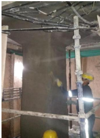
Figure 10: Showing member with fire protection coating after strengthening.
