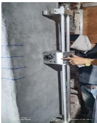
Figure 3: Marking the area to be strengthened
