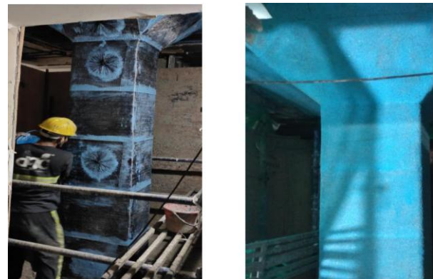
Figure 9: Showing fixing of carbon fiber anchors and top coat of our cafe.
