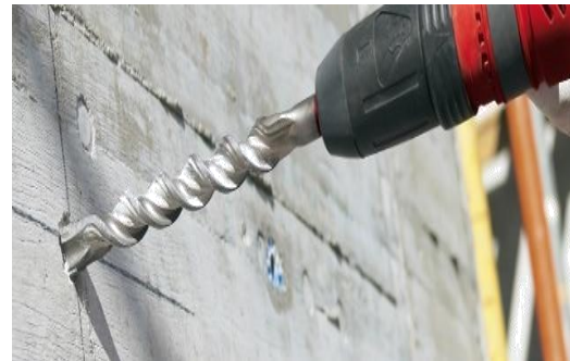
Figure 4: Drilling on concrete surface
