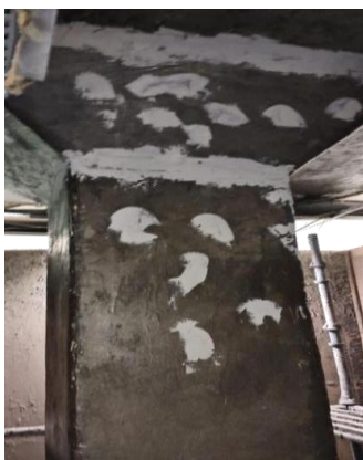
Figure 6: Putty application on the surface to be strengthened
