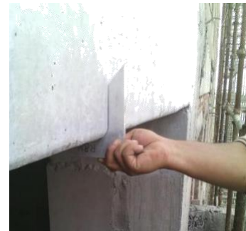
Figure 2: Checking the corners of the member with the Radius gauge
