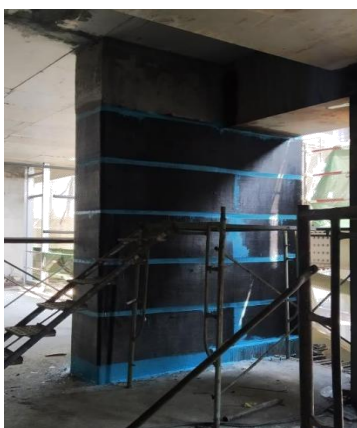
Figure 8: Showing the application of carbon fiber wrap
