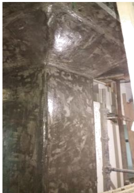
Figure 5: Primer application on the marked surface to be strengthened
