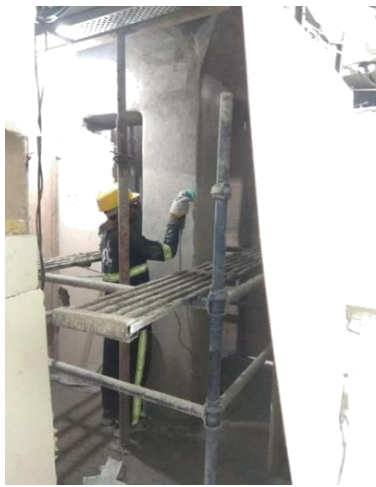
Figure 1: Removal of foreign deposits on the substrate surface
