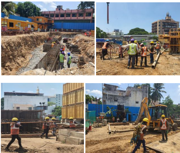
Fig -6 : Chennai Metro Rail Works ( Chetpet )
