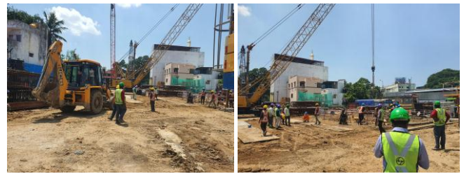
Fig -5: Chennai Metro Rail Works ( Purasaiwakkam )
